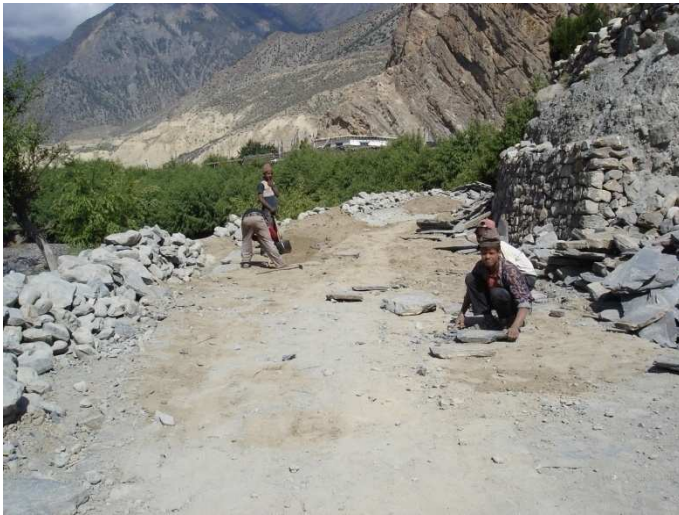
Photo 6. 8 Labourers are working on road construction in Mustang
