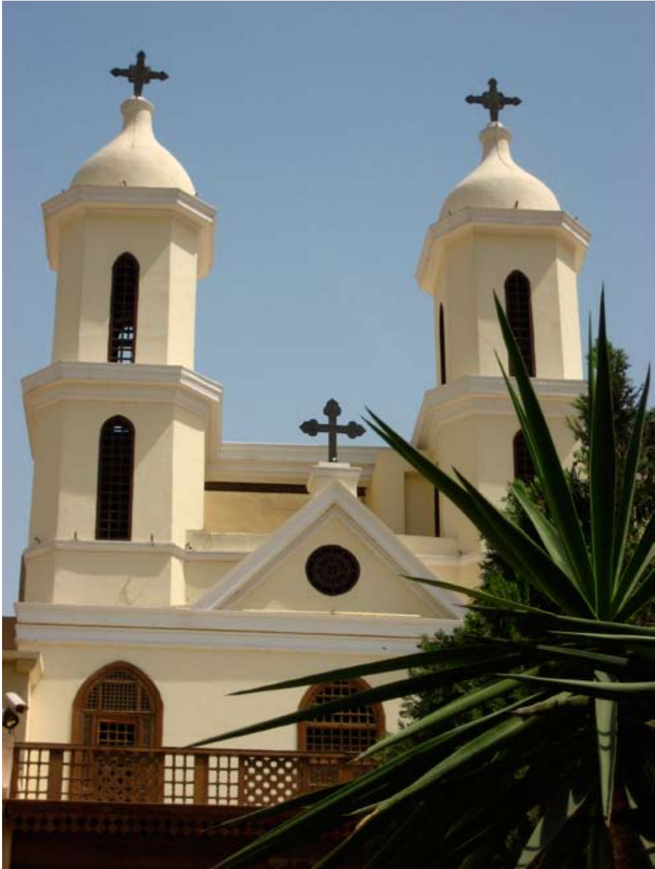
Fig. 3. Saint Virgin Mary's Coptic Church or the Hanging Church in Old Cairo built on top of the Water Gate of Roman Babylon. Photo: Terje Oestigaard.
