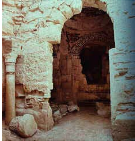
Fig. 7. The tomb of St Menas paradoxically at risk from the rising waters of the site.
