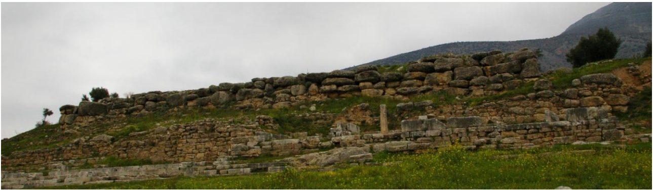
Figure 17: The retaining wall of the Old Temple Terrace (Photo: Patrik Klingborg)
