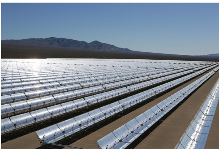
Figure F.3: A closer look at the parabolic troughs which collects the solar energy and focus it on the receiver tube filled with Heat Transfer fluid at the focal line. The location are Nevada solar one in Nevada, U.S [114]
