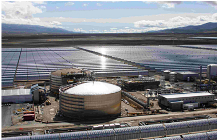
Figure F.2: A closer picture of the indirect two-tank storage system at Andasol. The system have a thermal capacity of 1050 MWh, enough for 7,5 hours of full load power production (50MW) [113]
