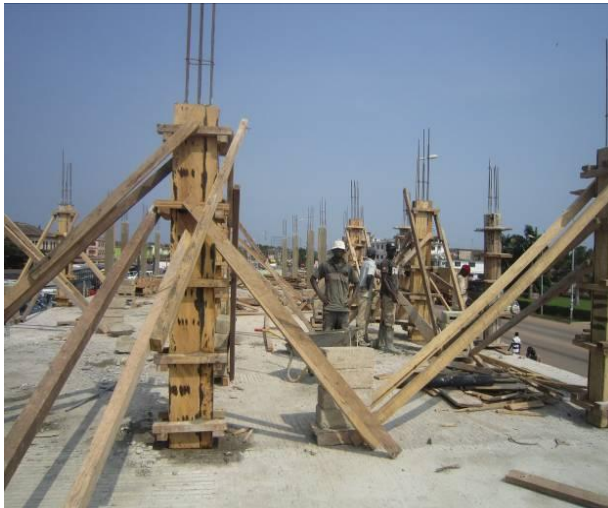
Plate 7: Supporting concrete with wood.
