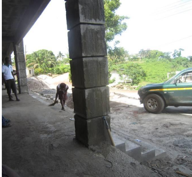
Plate 11: Woman sweeping construction site.
