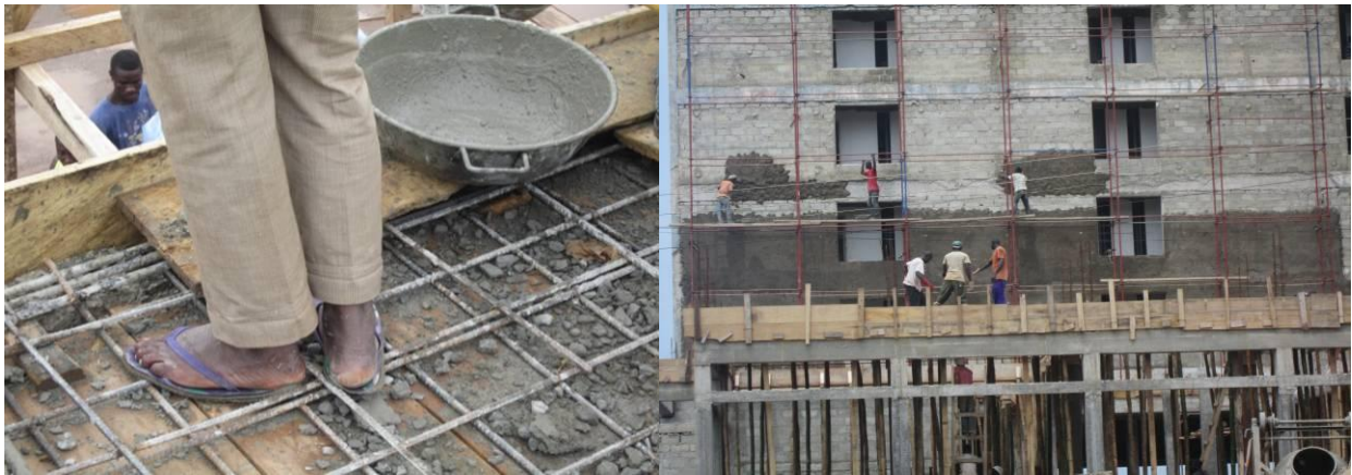
Plate 26: Standing on iron rod in bathroom slippers. Plate 27: Standing on wooding scaffold; only one person had a helmet on, another person extreme left had a hat on.
