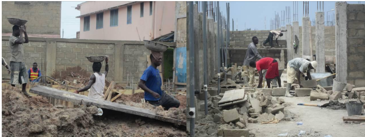
Plate 9: Casual workers carrying concrete.
