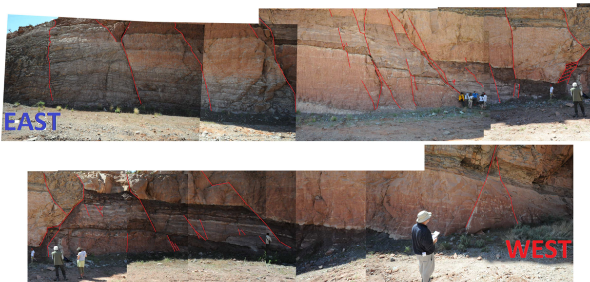
Figure 1-5 Image of the road cut south of Arches National Park (ANP) along highway 163 in southeastern Utah. The image is viewed from the north. The red lines indicate small faults in the hanging wall damage zone of Moab Fault, (not pictured, to the left of the top image). This image is a composite of photographs taken by Anita Torabi.
