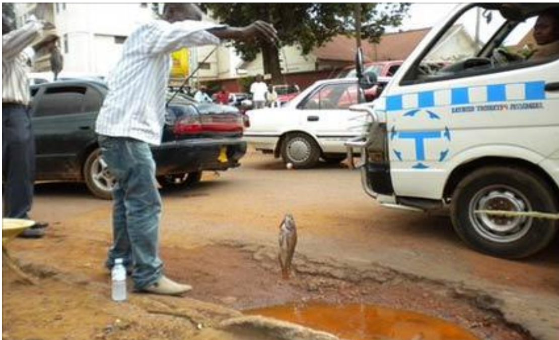
Figure 2: Are Kampala's potholes big enough to fish in?
