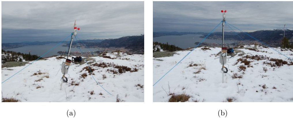
Figure 5.3: Tilted weather mast due to a broken pole at Strandafjellet Feb/Mar 2011 (a) before and (b) after repair on 17 Mar 2011.
