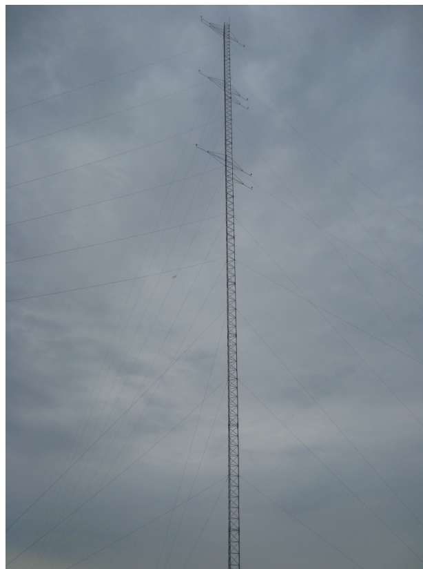
FIGURE 3.15: Meteorological Mast at Ona island (Source: Vestavind Offshore AS).
