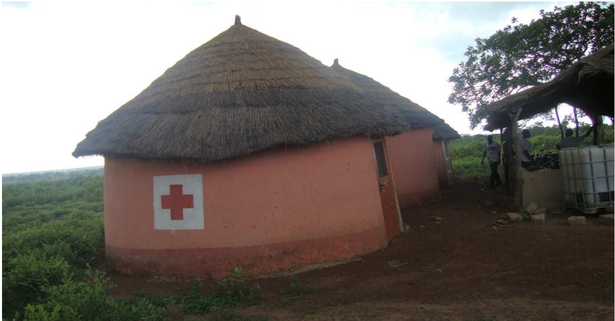
Figure 24: Health post provided by BioFuel Africa Ltd. Photo: Author, 2009.
