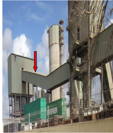
Figure 8: An enclosed conveyor belt system in the cement mill (Red arrow) (Photo by Tungu)
