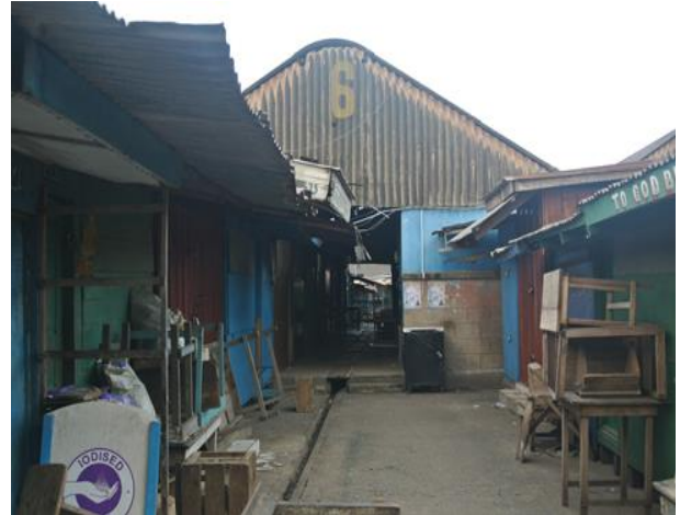
Photo 7. One of the eight sheds, Shed 6.
