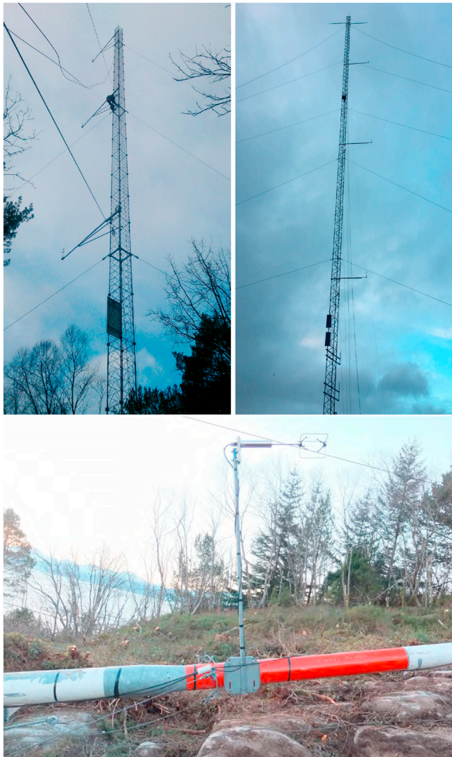
Fig. 4. Examples of mast structures used. Rectangular lattice tower at Aakvik in Halsafjorden (upper left), Kvitneset in Sulafjorden (upper right), and Halsanaset in Halsafjorden (below), where one of the anemometers can also be seen. Photos: Kjeller Vindteknikk.
