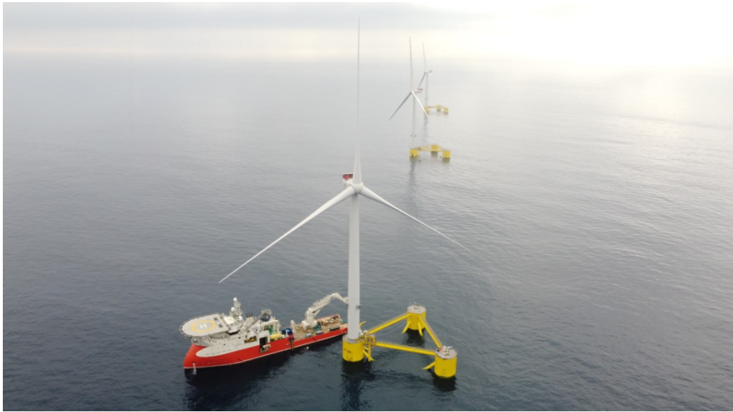
Figure 2.7: The picture shows three wind turbines in the WindFloat Atlantic wind farm outside Portugal. All three wind turbines are installed on Tension Leg Platforms. Picture from EDP (2022)
