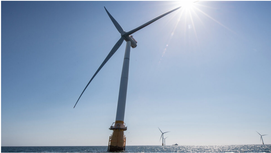
Figure 2.4: Five SWT-6.0-154 are used in Hywind Scotland, the first commercial floating wind farm ever to be built. Here represented by a SWT-6.0-154 from Hywind Scotland. Other turbines from the farm can be seen in the background. Picture from Wind Europe (2022)
