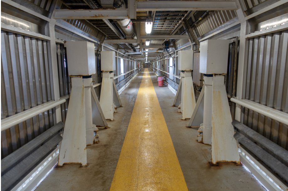
Figure 3.3: Housings of the four laser altimeters in the LASAR instrument, located on the footbridge connecting the Ekofisk 2/4 B and 2/4 K platforms. Photo by the author.
