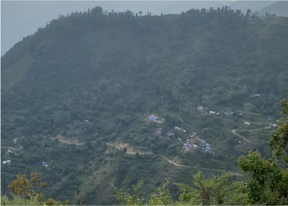
Figure 5: Feeder-road available for transportation access to the Chepang community
