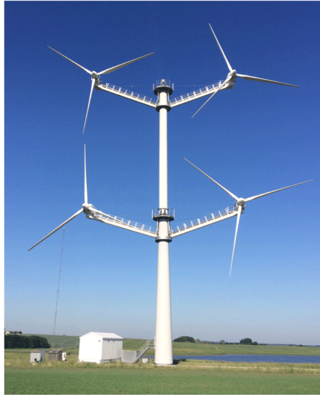
Figure 1.1: Vestas multi-rotor demonstrator. Each rotor has a diameter of 29.2 m, and the tip spacing is 1.82 m. Retrieved from [15].
