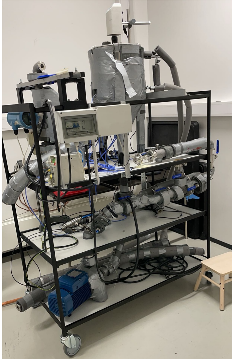
Figure 3.5: The flow loop under construction. Visibly, there are several open ends in the piping.
