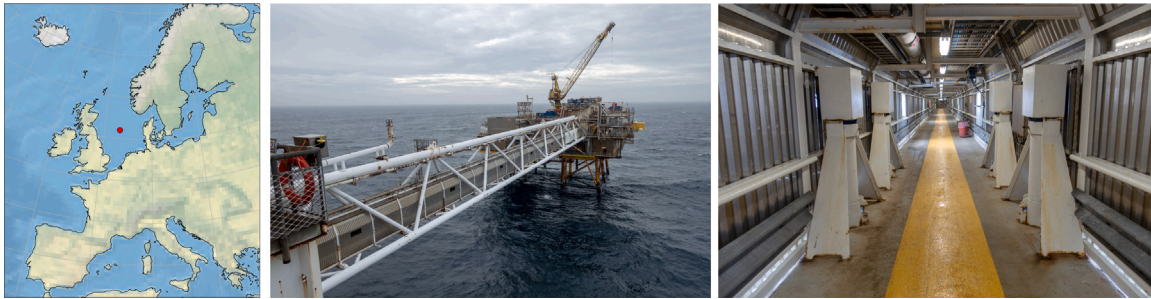
Fig. 1. Left: Ekofisk location in the central North Sea marked by the red dot. Center: Footbridge between the Ekofisk 2/4 K and 2/4 B platforms, looking toward the 2/4 B platform. Right: The 4 laser altimeters placed in a 2.6\text{ m} \times 2.6\text{ m} array formation inside the footbridge.
