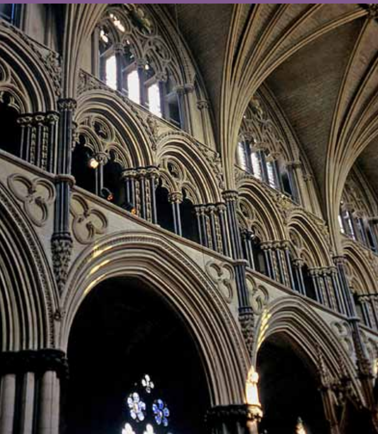
Fig. 7. Purbeck marble shafts at the Angel Choir in Lincoln Cathedral. Photo: P. Storemyr
