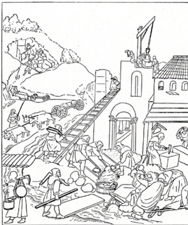
Fig. 6. Lay brothers building the Cistercian abbey of Schönau in Germany, showing the process from quarry to masonry. Schönau was founded in 1142, four years before Lyse. After a pen-and-ink drawing from the 16th century, Germanisches Nationalmuseum, Nürnberg. After Du Colombier, 1973:48 and France, 2012: 55
