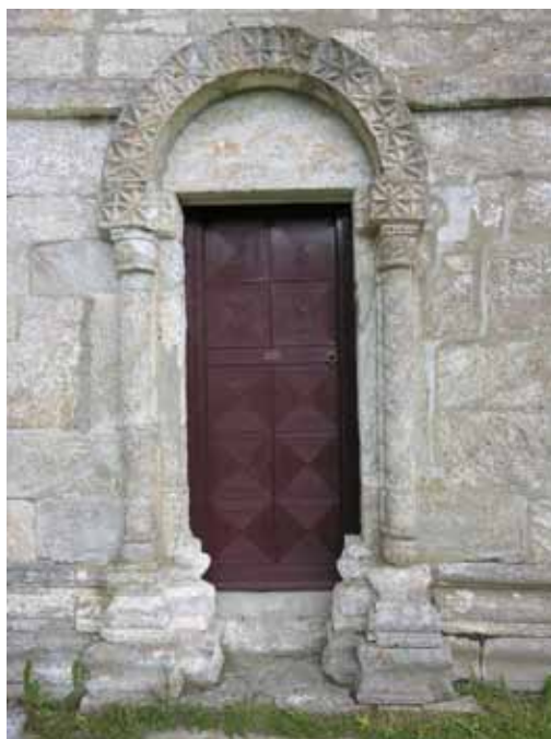
Fig. 4. The oldest part of the Alstahaug Church is built from soapstone ashlars. A round arch of soapstone with a carved pattern of «sunken stars» is seen over the choir door to the south. The Baroque poet Petter Dass was a clergyman here at the end of the 17 th century and until his death in 1707. Photo: B. Berglund
