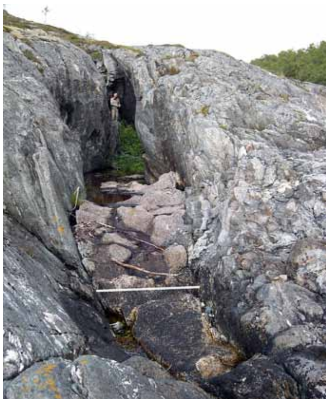
Fig. 7. Exhausted soapstone quarry at Haltøy, Nordland. The cavity defines the extracted volume of the original soapstone deposit. White line represent ancient shoreline by the time of quarrying. Photo: T. Heldal
