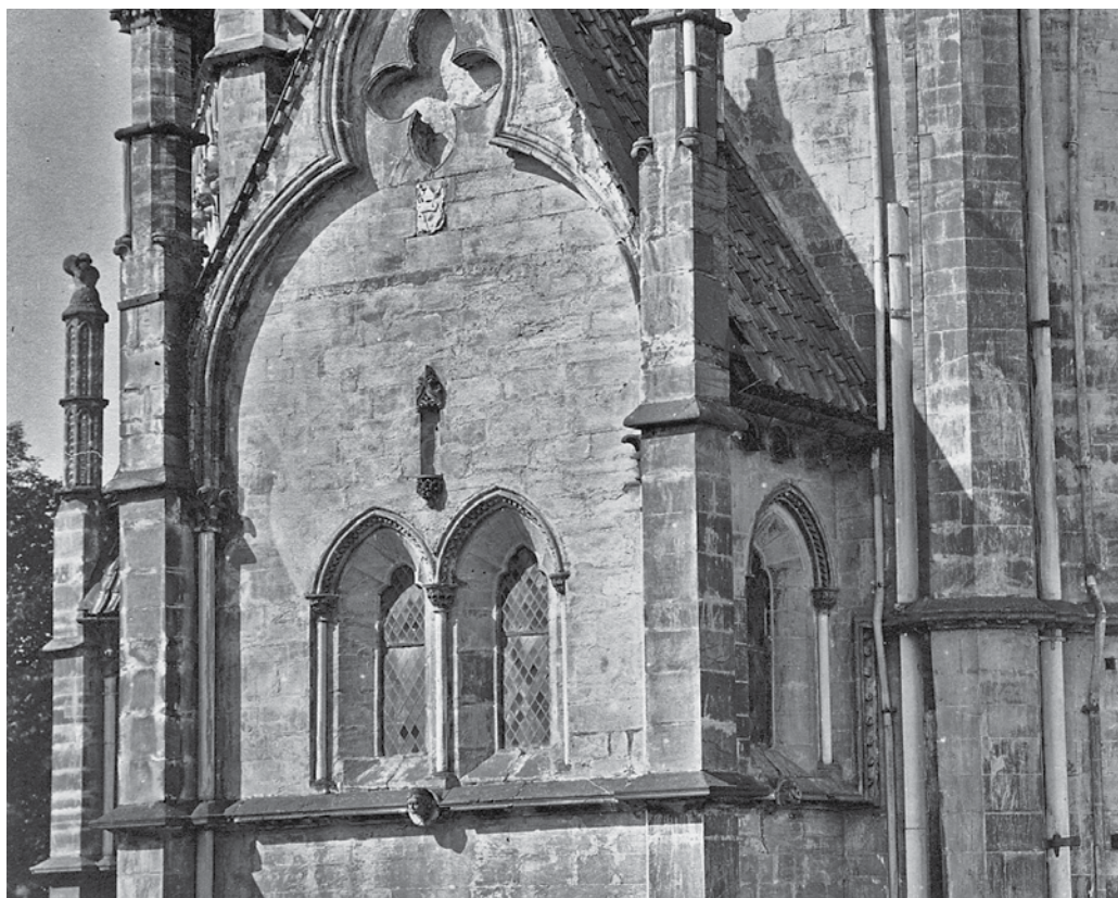
Fig. 2. Remaining marble shafts at the east chapel of the octagon at Nidaros Cathedral immediately prior to restoration in 1871. Most shafts are from Lænn in Sparbu. Photo: The Restoration Workshop of Nidaros Cathedral (detail of larger photo)
