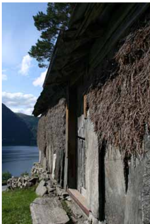
Fig. 7a. Barn wall covered by juniper ( Juniperus communis ) at the farm Havrå on Osterøy in the fjord area. Photo: B. Helle
