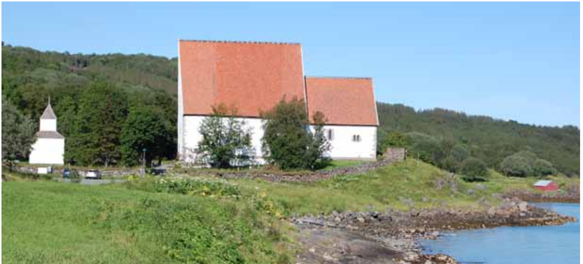
Fig. 6. View of Trondenes Church taken from the south. Photo: S. Wickler
