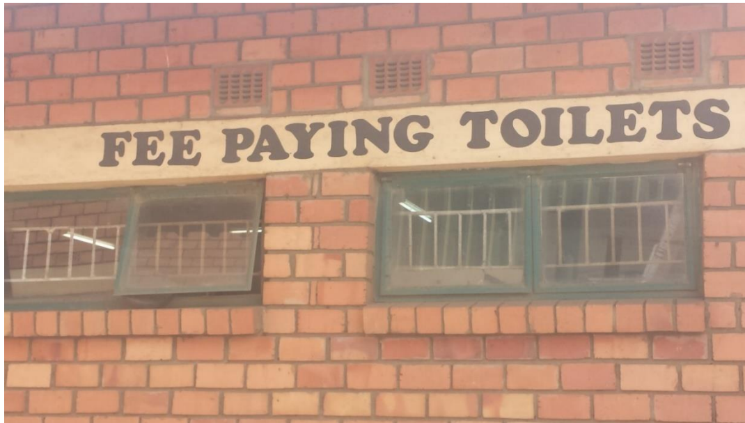
Image 6: Sign for fee paying toilets at a visited central business market. Traders at all markets had to pay for using the welfare sanitary facilities.
