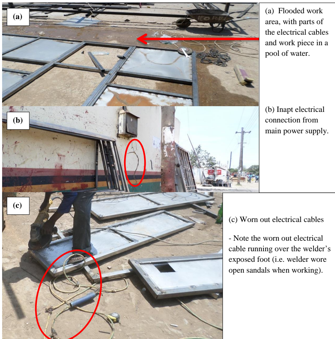
Figure 9: Electrical Hazards Observed
