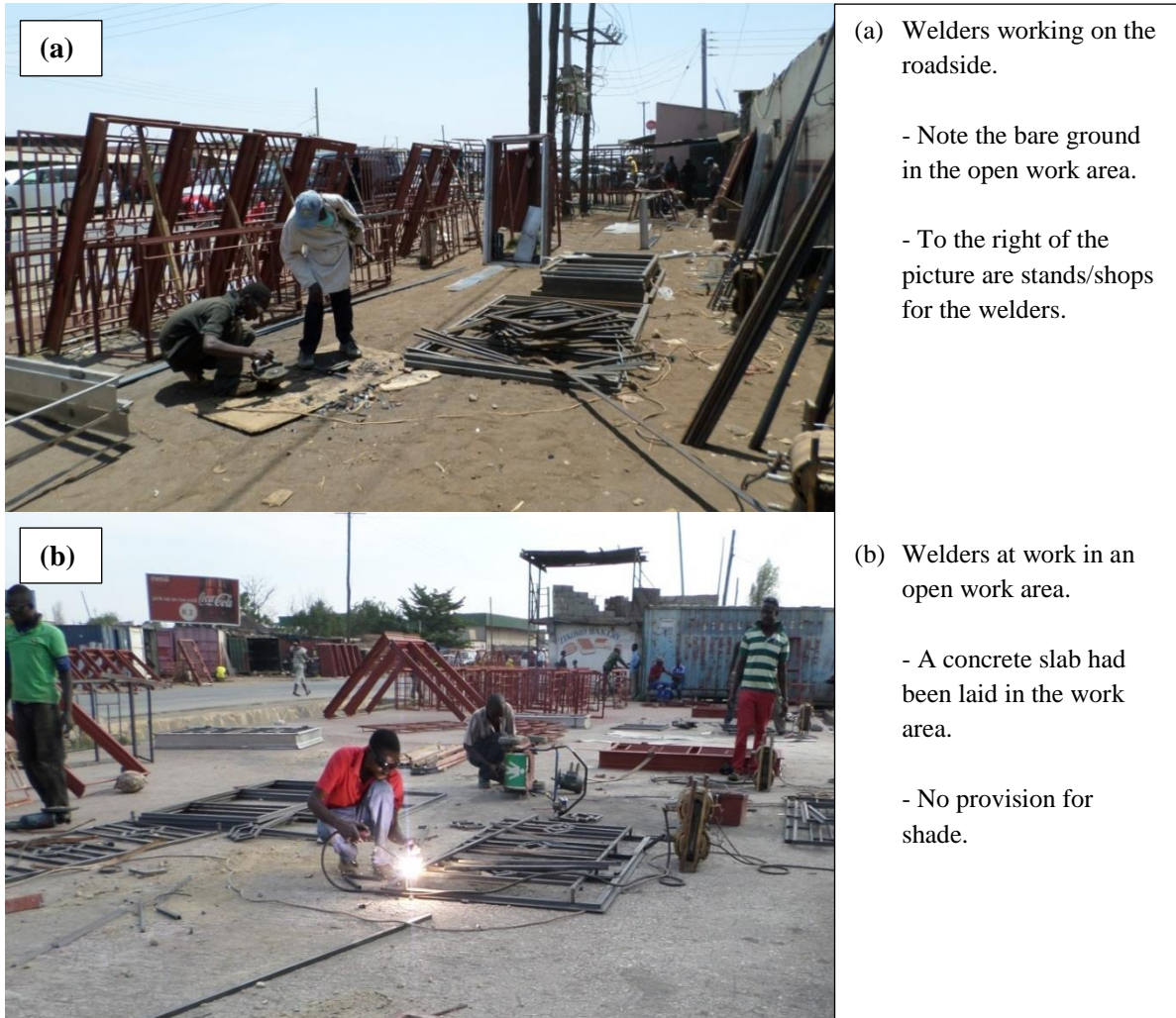
Figure 2: Work Areas for Welders
