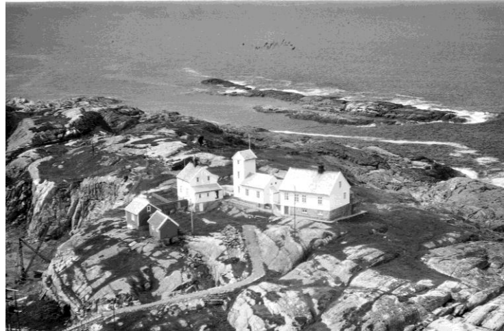
Figure 4 A old picture of the lighthouse on Møøya.
