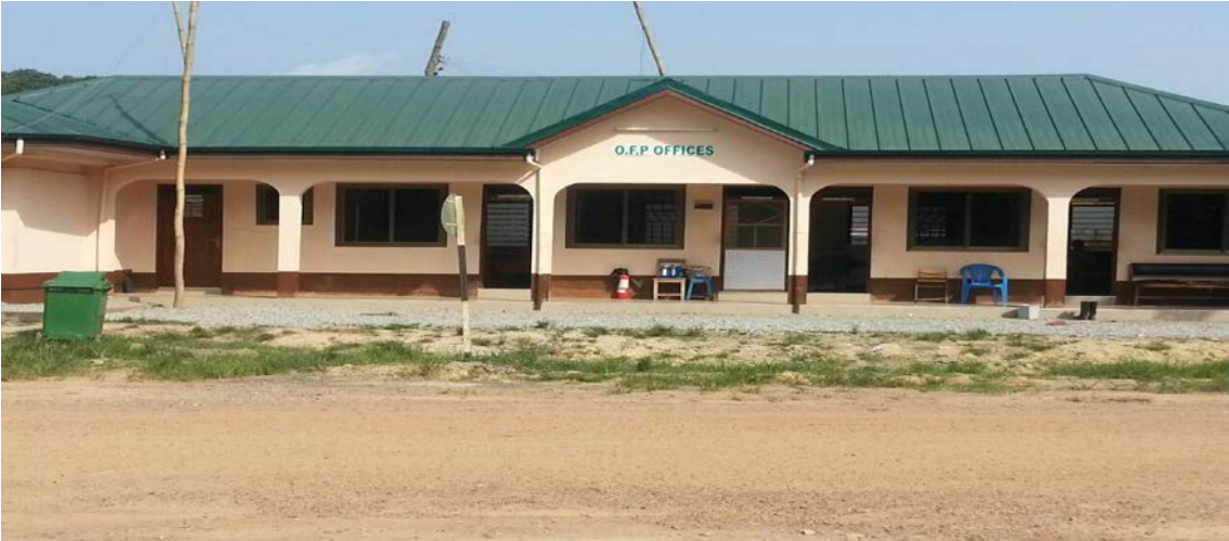
Photo 6: Newly constructed outside fruit purchasing offices at Norpalm
