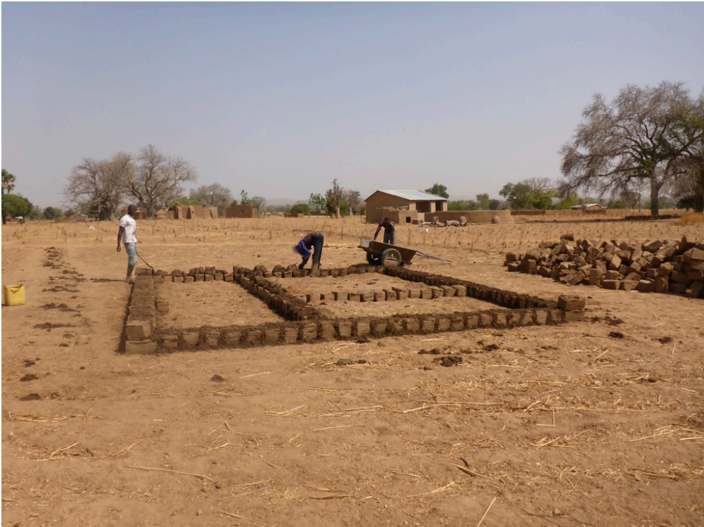
Local farmers are laying a foundation for a new house.
