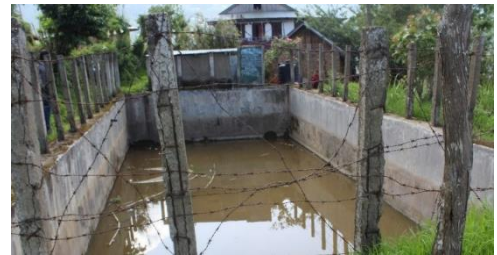
Picture 7.1: Water reservoir in Aahale
