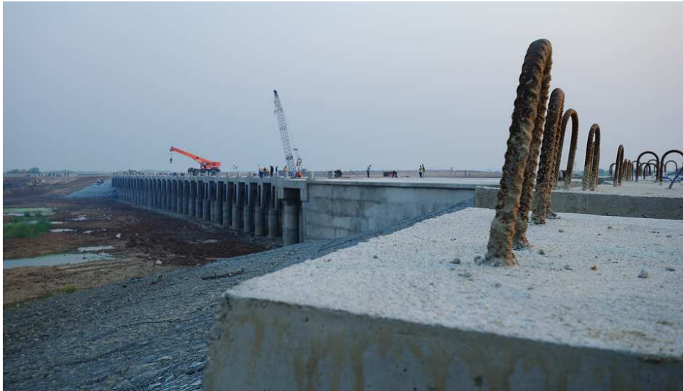
Photo 4. Nsanje River Port unnder construction in the Shire Valley, Malawi. September 2010
