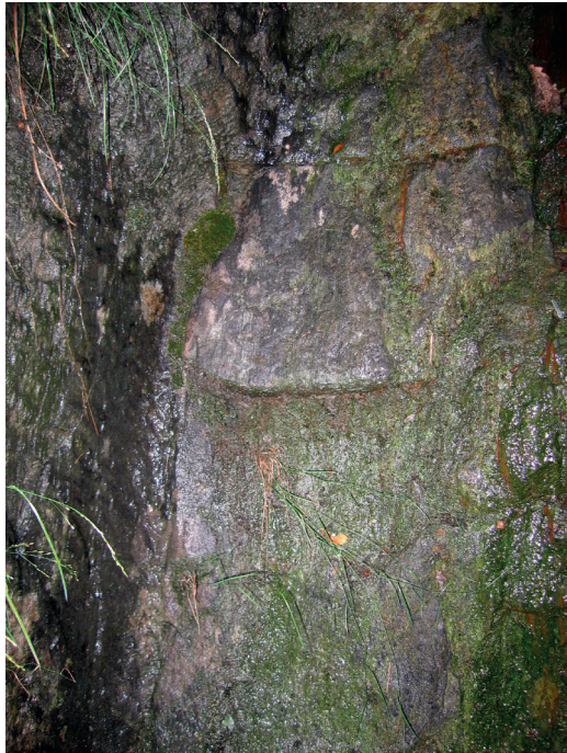
Figure 2. The soapstone quarry at Lyse. One can see traces of exploiting the quarry for ashlars. (Photo: A. T. Hommedal).
