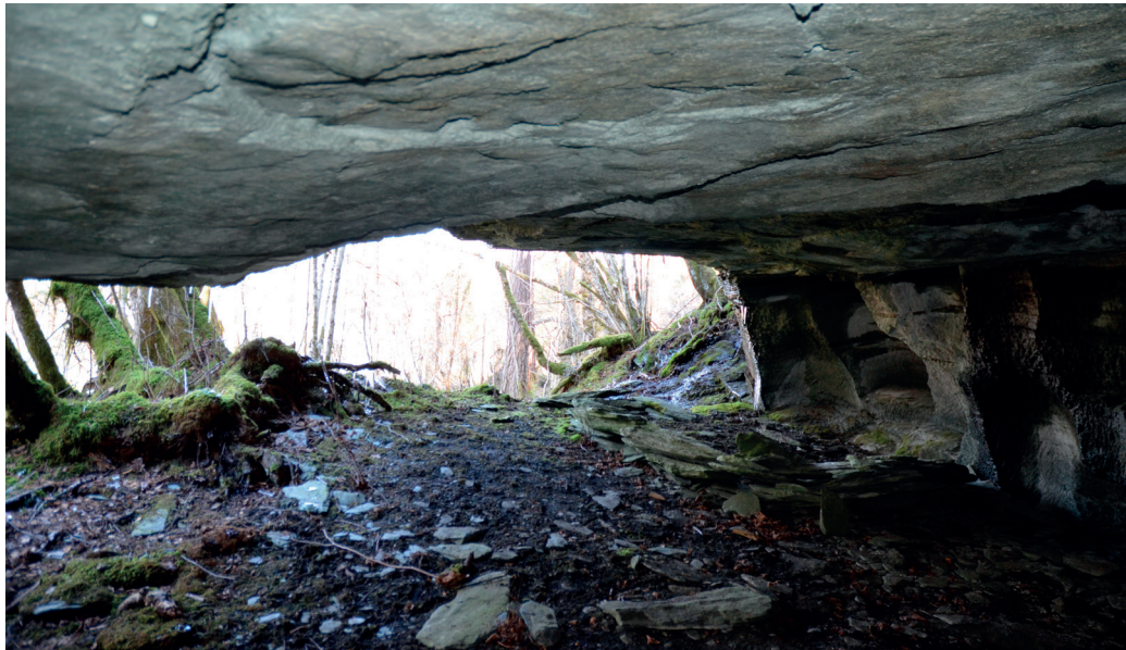
Figure 3: Underground quarry at Fugleberg Farm in Ølve. Production marks of bakestone extraction are visible on the wall to the right (Photo: A. O. Martinussen, 2012).
