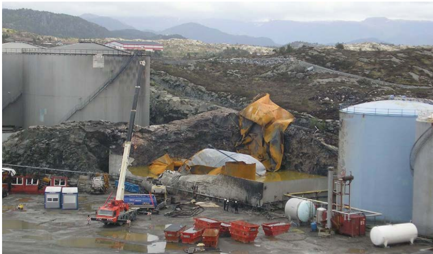
Figure 5: The land around the explosion site was partly covered with the sulphurous waste from the destroyed tanks. Photo taken before start of the clean-up operation. Photo: Glenn Rogers, M/T Karen Knutsen, Knutsen OAS Shipping.
