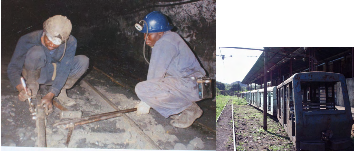
Fig. 6. Underground transport worker fixing rail lines (photograph by Simon H.D. Mamuya)
