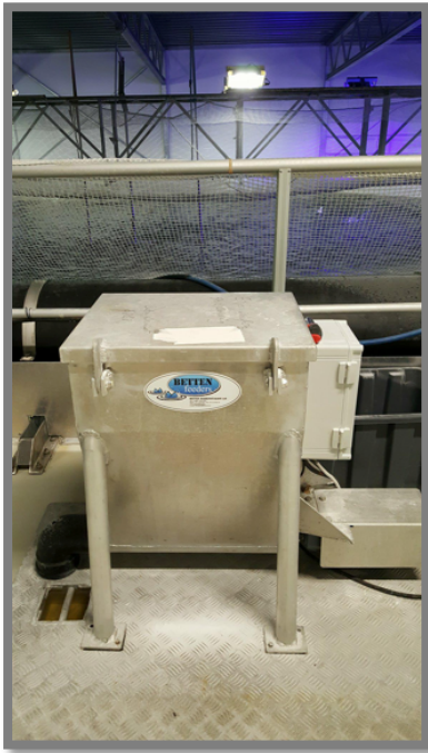
Figure 8: Dosing tank for bicarbonate, releasing powder into the biofilter. Photo: Karine Drønen
