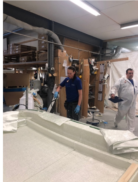
Picture 6. Preparation for vacuum [31]
