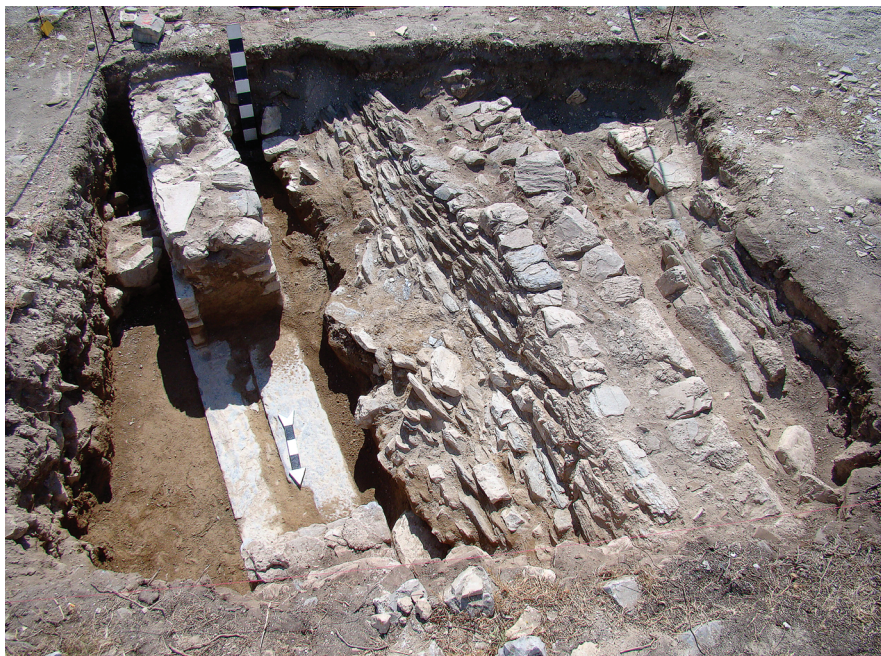
Figure 15. The collapsed vault of the narthex.
