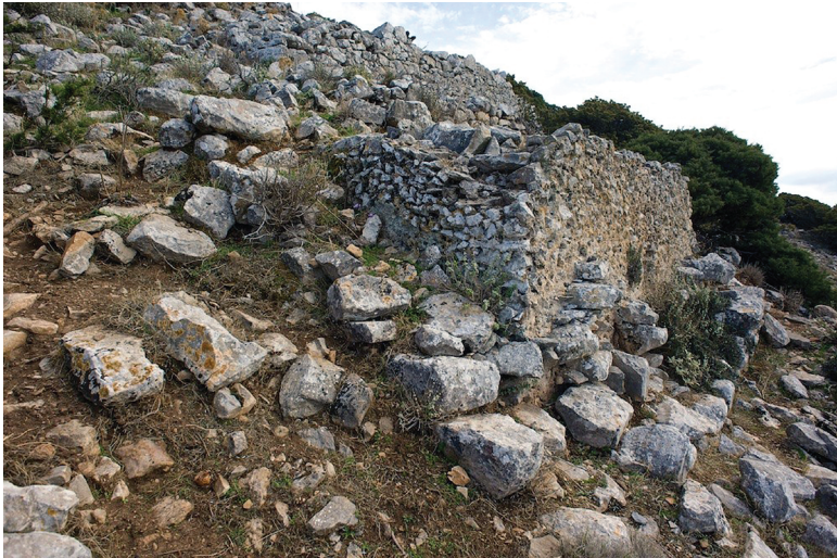
Figure 11. Terrace supporting house with cistern, below, and narthex of church, above.
