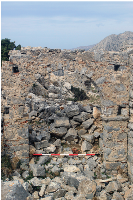
Figure 5. Arch inserted into the main aisle of Building A.
