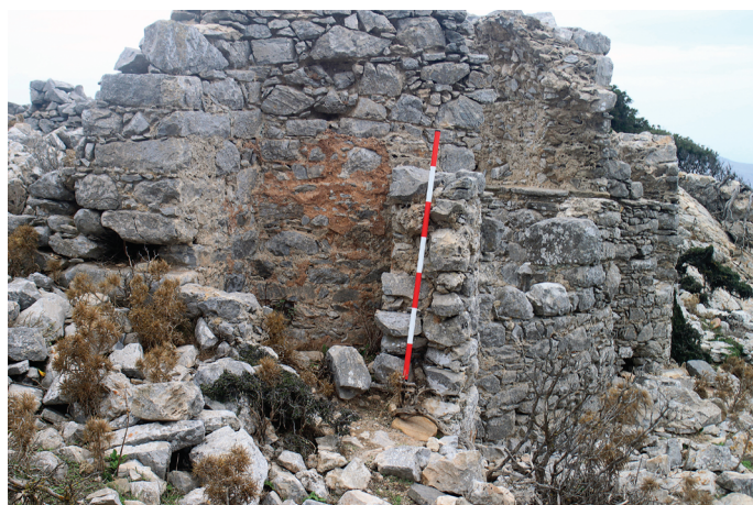
Figure 7. Eastern facade of Agios Georgios seen from the south, with the small cistern in the foreground.
