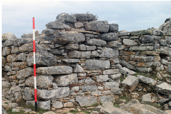
Figure 6. Northwestern corner of Agios Georgios complex (buildings D and C).
