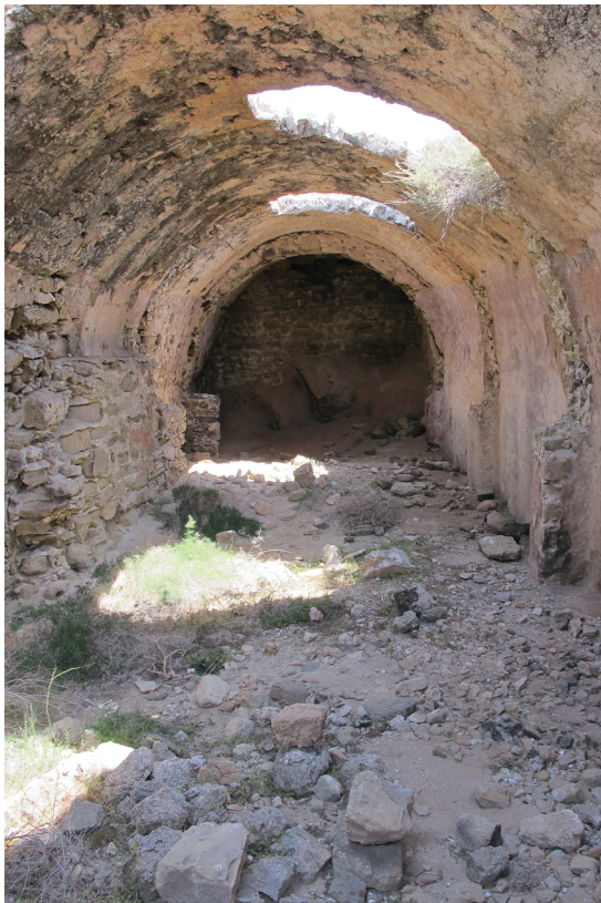
Figure 8. Interior of Cistern BB-3.
