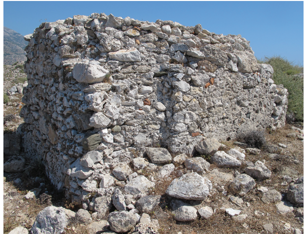
Figure 7. Cistern B03 (from southeast).
