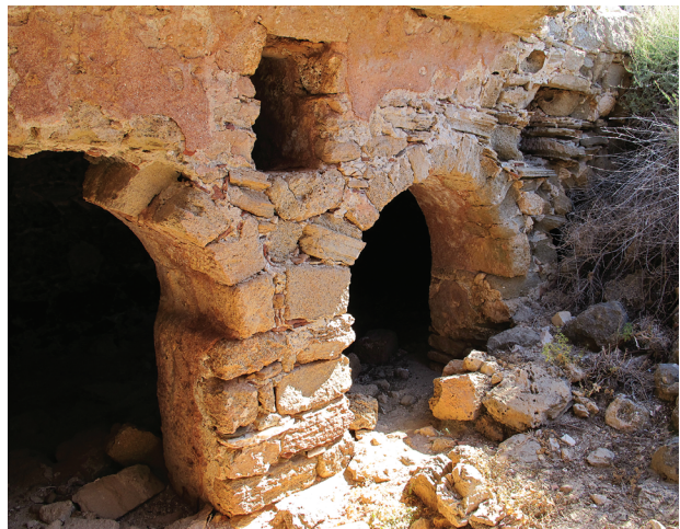
Figure 9. Interior arcade of Cistern AA.
