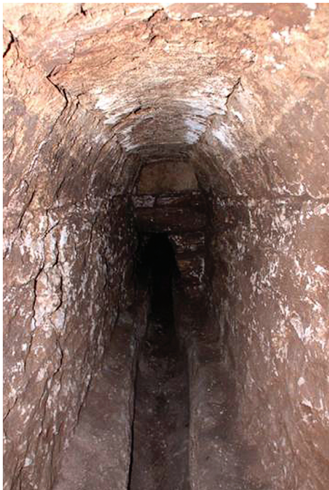
Figure 5. Vaulted corridor at the Roman entrance to the tunnel of the aqueduct in Melanes.
