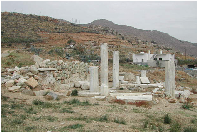
Figure 3. Agios Stephanos. View from E. Before restoration programme.
