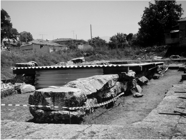
Figure 8. Temporary protection shed for the excavated area in the temple trench, after the 1992 season. (Photo: Nordquist)
