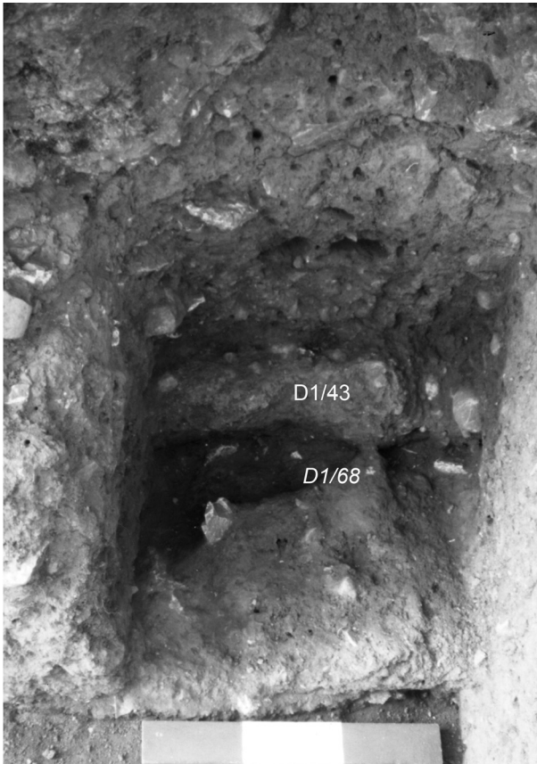
Figure 29. Part of the south wall of Building 1 in square D1 (unit D1/43), with part of the large posthole D1/68. (Photo: Nordquist)
