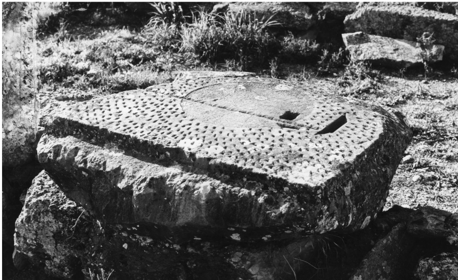
Figure 21. Stylobate block on the southern colonnade foundation, with markings for the wooden column and for the plug securing the column in its correct position. (Photo: Østby)
