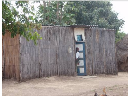
Picture 2. Valley house
