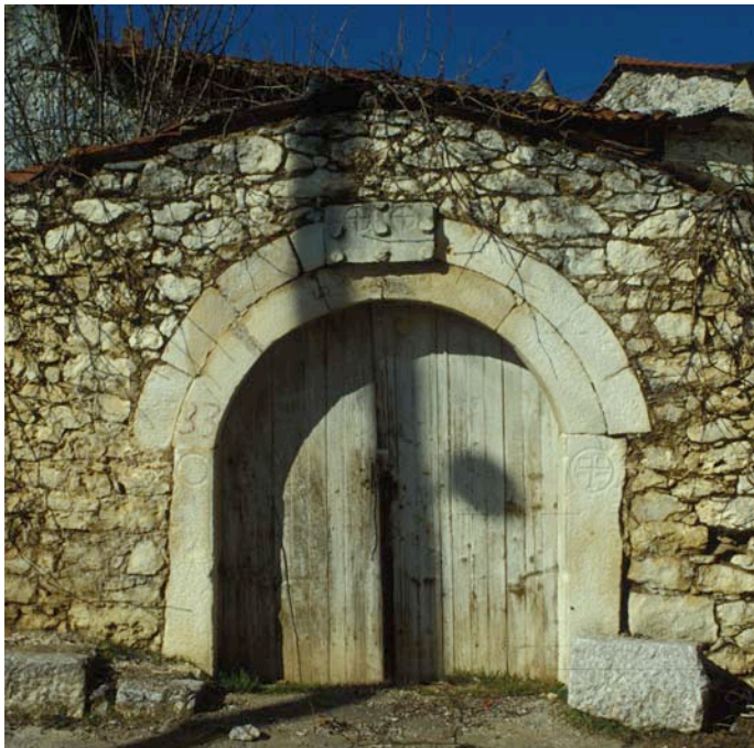
Figure 3.6 Monumental guttae fragment inserted as a key-stone in the arched gate of one of the village houses at Lithovounia.
