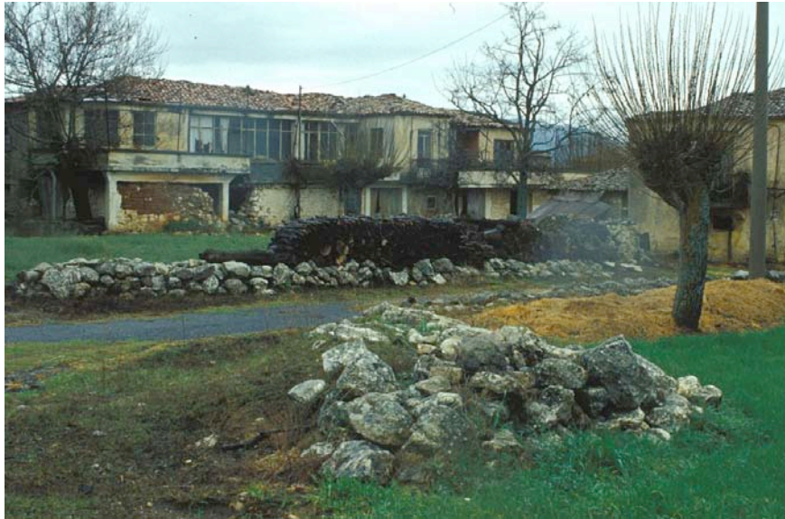
Figure 4.27 Ruins of the 'old tower' at Pirgeïka.
