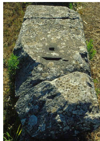
Figure 2.4 One of the four in situ stylobate blocks with markings from the interior wooden columns in the cella of the archaic temple in the sanctuary of Athena Alea.
