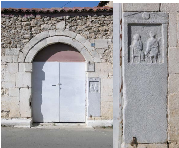
Figure 4.26 Gate of an old village house in Stadio. An ancient spolium is built into one of the pillars in the gate as a decorative element. Detail of an ancient stele on the right.
