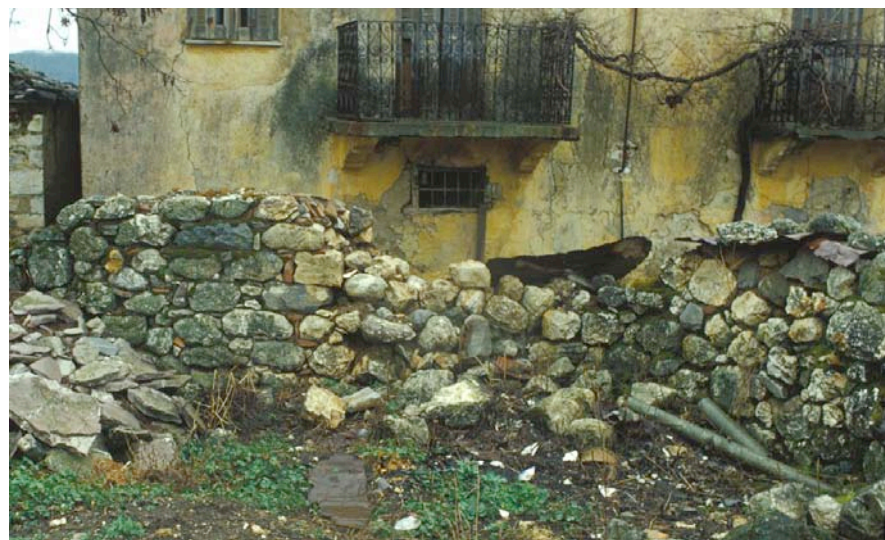
Figure 4.31 Early modern masonry technique in the 'old tower' at Pirgeïka.
