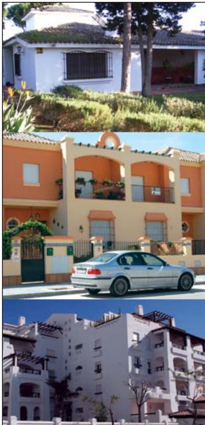
Housing on the economy can be in single family homes with yards, townhouses or high-rise apartments.
