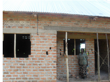
After Joining NAADS-house under construction
