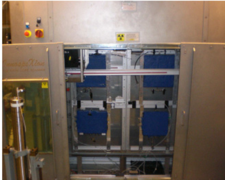
Figure 4-2: Four slabs mounted in the scanner cabinet. (Noremark, 2010).
