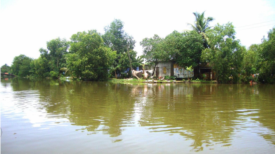
Fig.6. Partially submerged houses at the time of floods in Lower Kuttanad.
