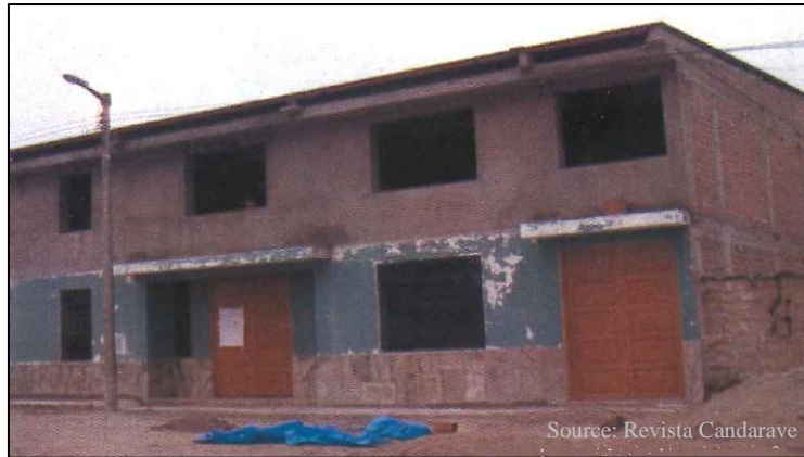
Figure 7: Huaytire Municipality building under construction
