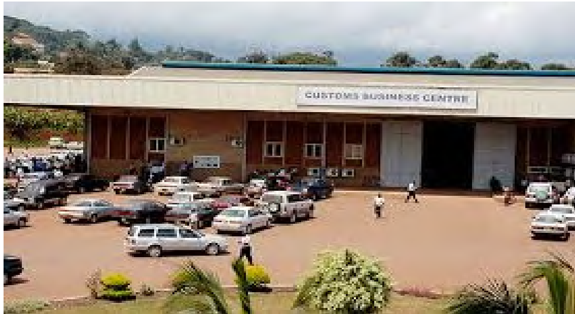
Figure 5: Customs Business Centre at URA headquarters in Kampala Uganda
