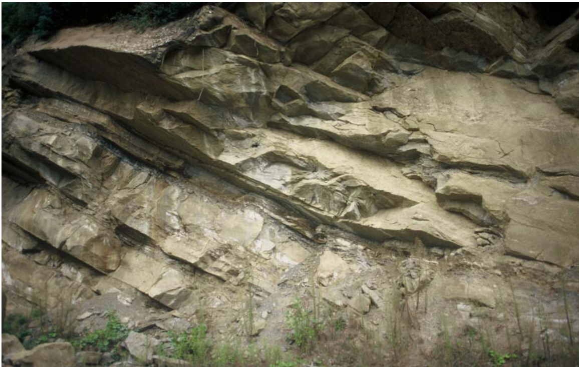
Figure 3.2. Sandstones of subfacies F2a, stacked directly upon one another and to various degree amalgamated (example from the lower part of Gürsöku Formation; see Log 1a in Appendix 1). The stratigraphic thickness of the exposure is ca. 6 m, and the way up is to the upper right.
