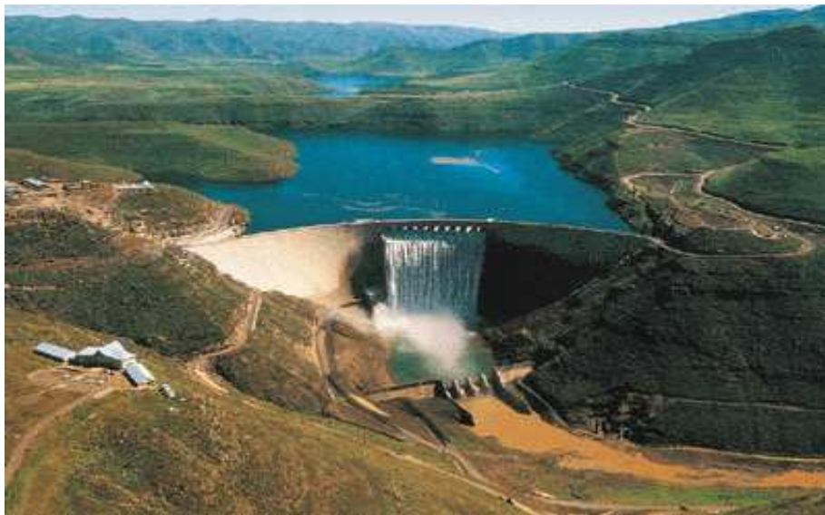
Picture 7: “The Katse Dam”. Located on the Malibamatso River in Lesotho, the Katse Dam is 185 and has a storage capacity of 1950 million m 3 (Picture: TCTA).
